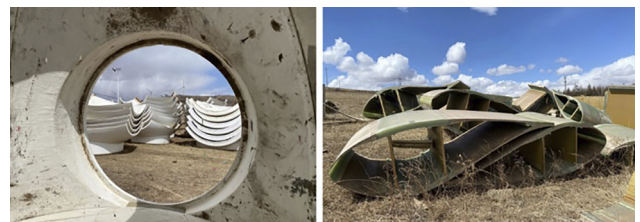
Fig. 2. Dismantled and cut end-of-life wind turbine rotor hub and blades, with large number of working wind turbines in the background (Photo by M. Wang)
